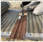
All anchors are provided with the mat. Depending on your mats' dimensions, the number of eyelets and anchors will be different
