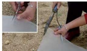
**Step 1:** Prepare the Mobi-Fence™ at the expected length (cauterize the fabric with a soldering iron in order to avoid the raveling)
